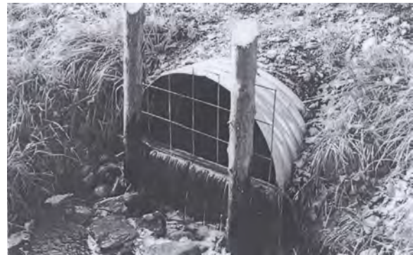
Figure 4. Dam board on culvert outlet
