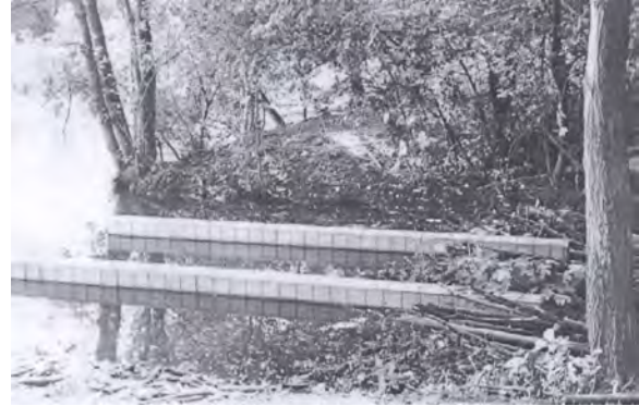
Figure 6. Wooden pipes installed in a beaver dam
