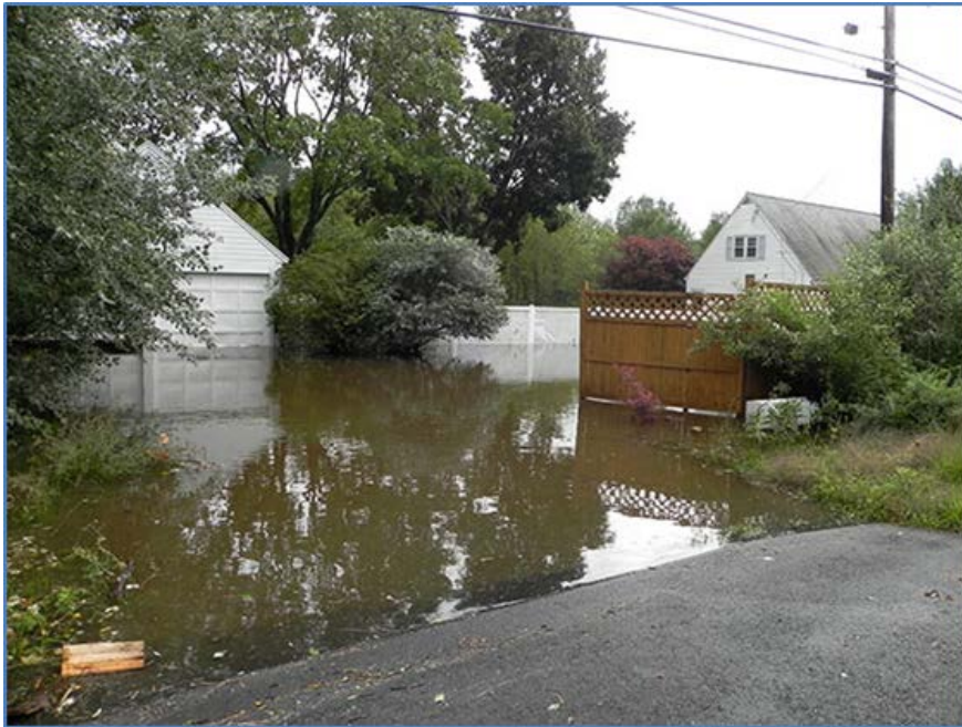
Figure I.2: Flooded home on Litchfield Turnpike after Hurricane Irene.
